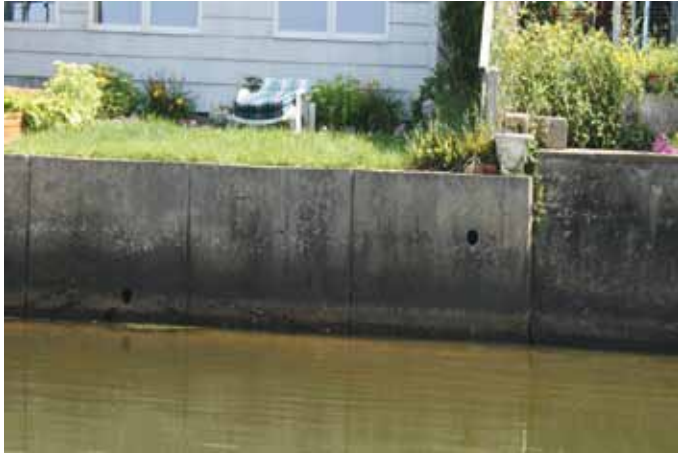
Retaining walls have been a historic remedy for eroding shorelines (note the storm-drain outfall pipes).
